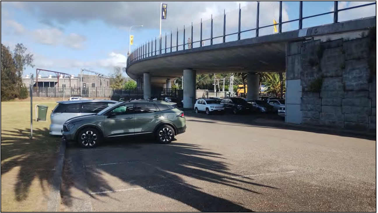
Photo P1-9: Car park, and Brian McGowan Bridge overhead.
