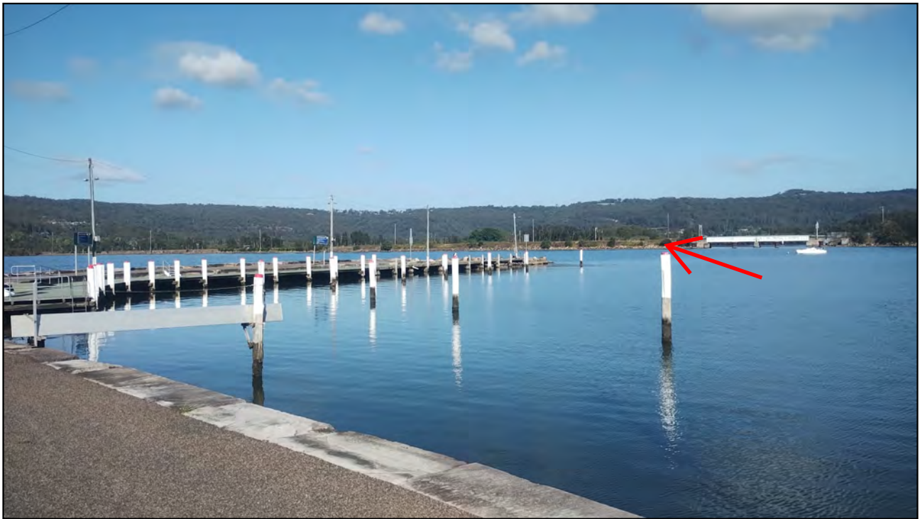
Photo P1-1: View from Gosford Public Wharf. Train line in the distance (arrow).
