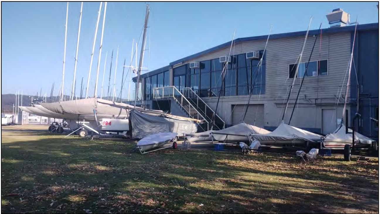
Photo P4-5: Gosford Sailing Club (southern side).
