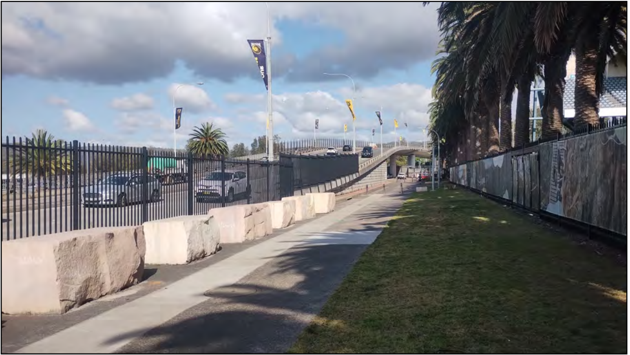
Photo P2-1: Brian McGowan Bridge in the distance.
