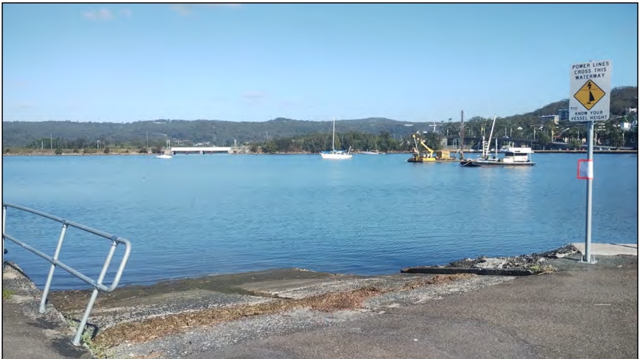
Photo P1-14: Boat ramp.
