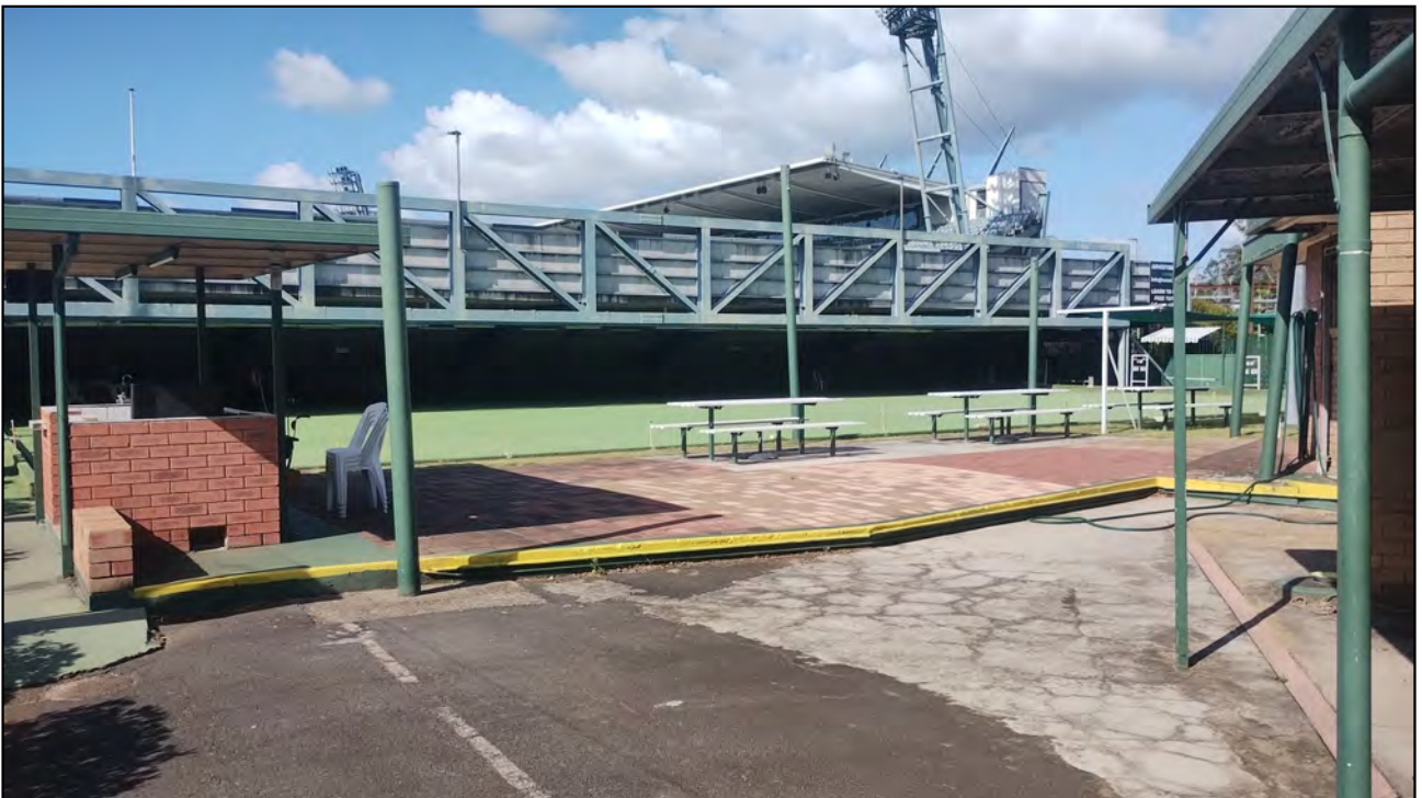
Photos P2-8: Western portion of Gosford City Bowling Club.
