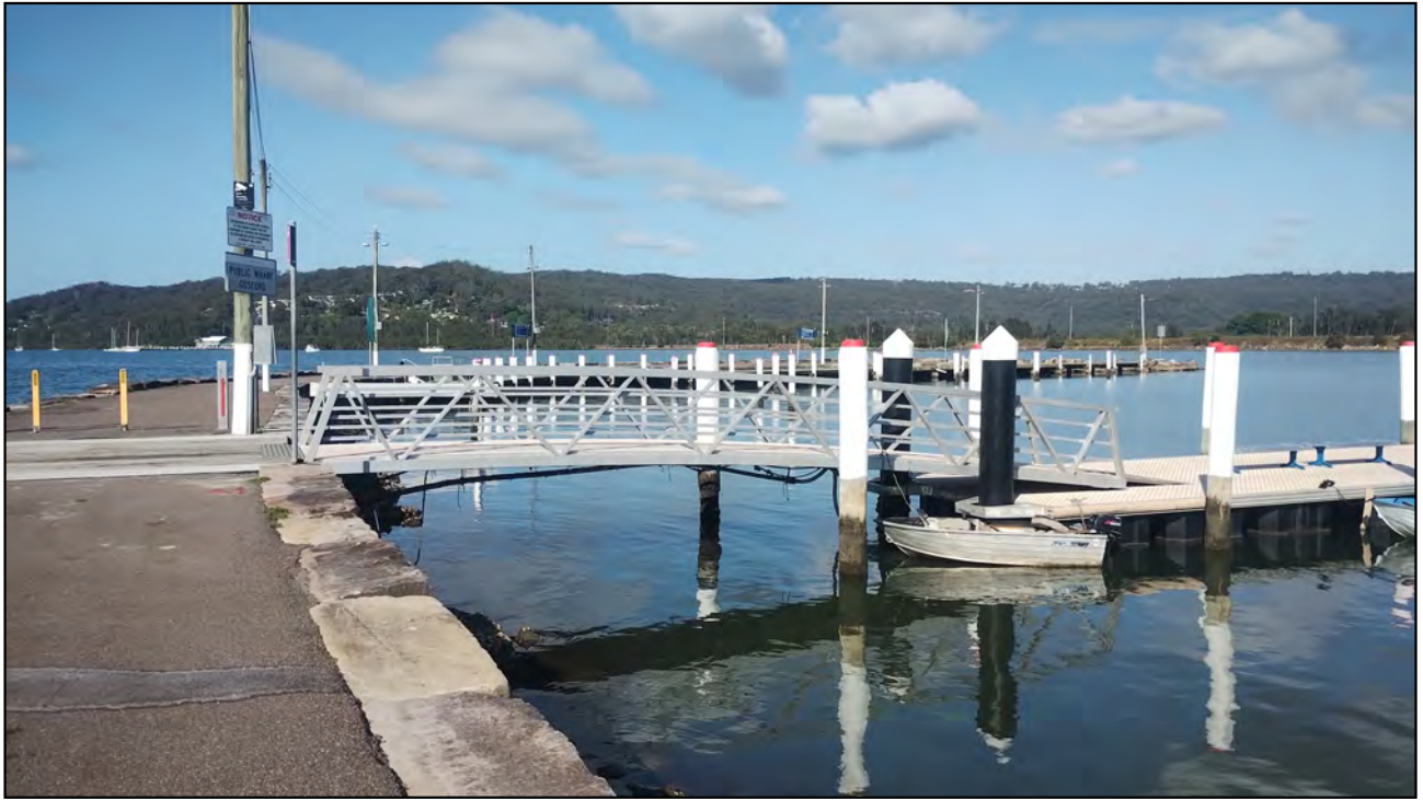
Photo P1-13: Breakwall / Gosford Public Wharf.
